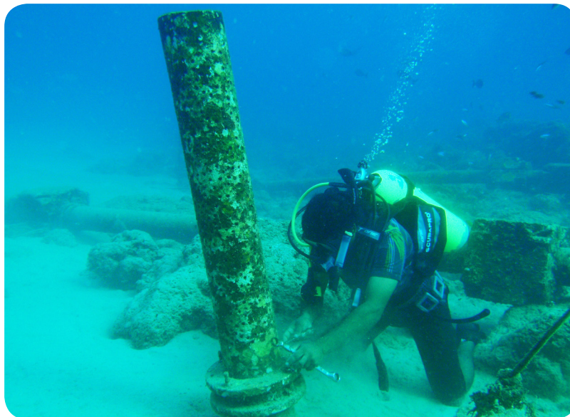
Maintenance of the seawater intake pipeline of the grouper project being carried out
